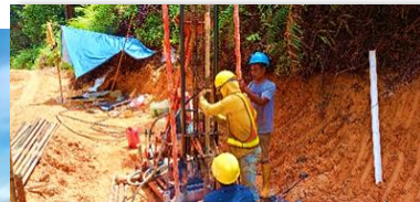
Drilling for sampling
