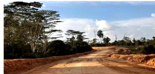
Portion of completed hauling road
