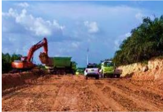
Land clearing for hauling road
