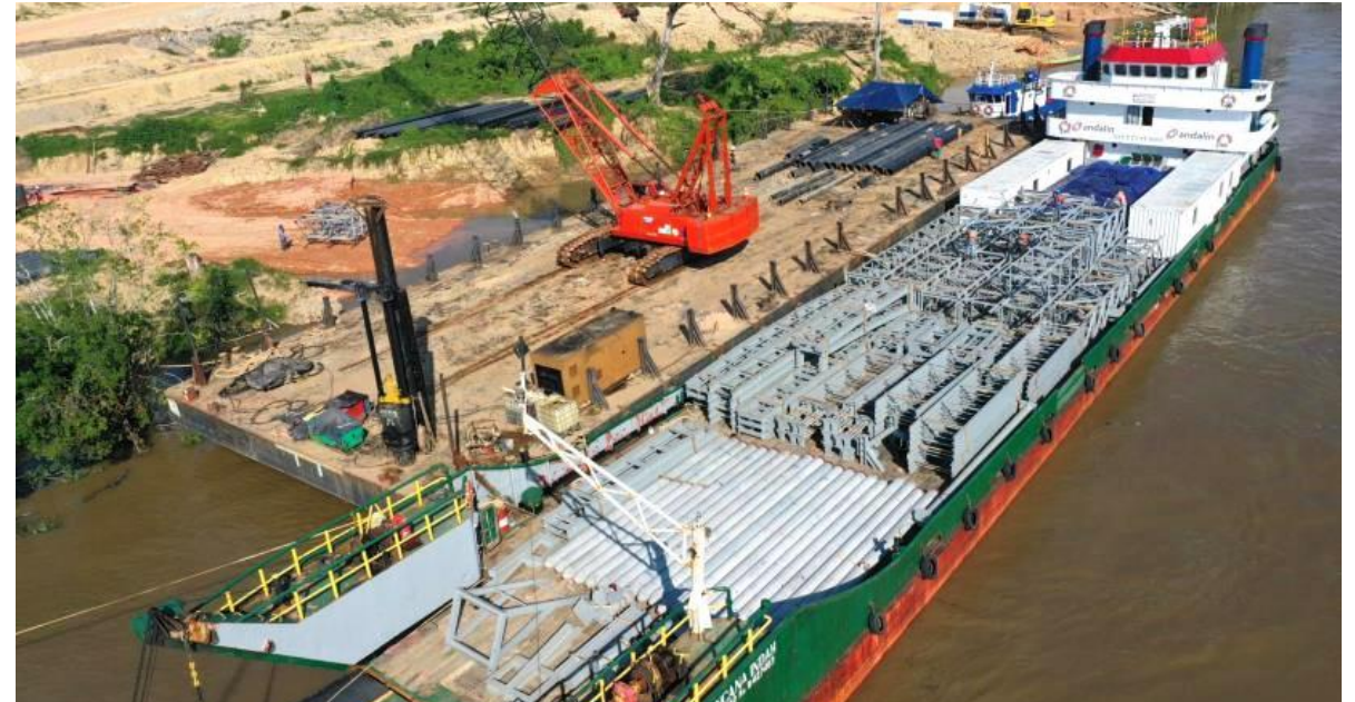
Material delivery for conveyor construction
